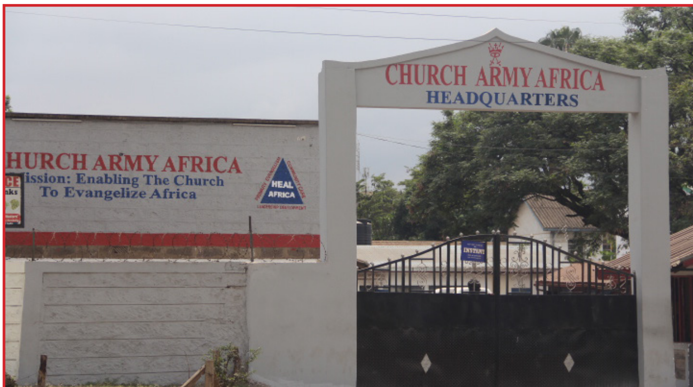
The shape of the new gate
